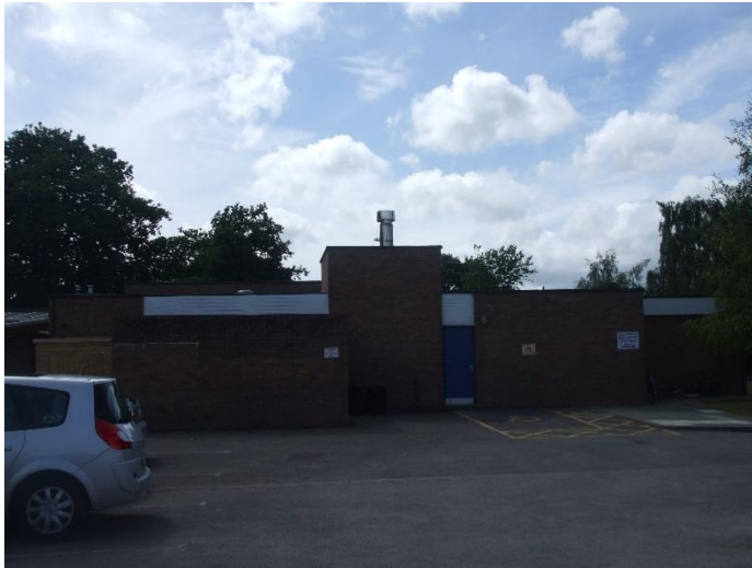
Side Elevation (Car Park)
